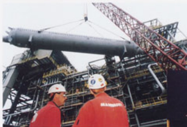
Dunkerque/Geleen - A 240 tonne pool reactor and other equipment were transported from the factory in France to the DSM chemical plant in Geleen over land and by water. At the Urea plant UF2 FSM Geleen project, Mammoet's 400 tonne lattice boom crane with superlift attachment took care of the lifting and positioning.
